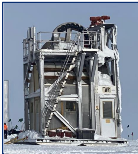
Installation of 6 strings at South Pole in 2026
